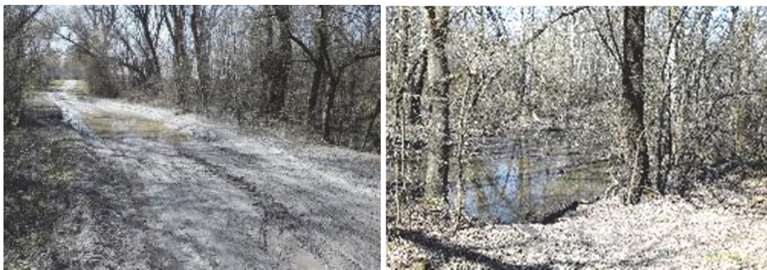
Figure 4.29 Problematic dirt road with a spillway crossing a stream without a culvert
