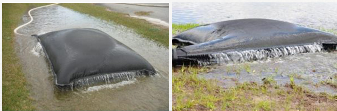
Figure 5.1 Proposed solution for the drainage of sediments and organic ( https://spillcontainment.com/products/ultra-dewatering-bag/ )
