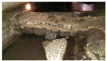
Figure 9 Missing capturing device on overflow edge
